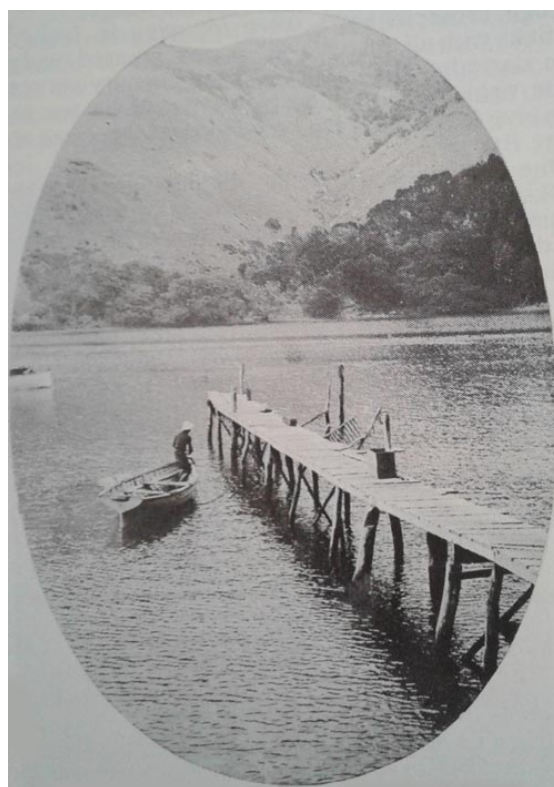
A typical Barrier jetty. Tea-tree lasted well in salt water.
